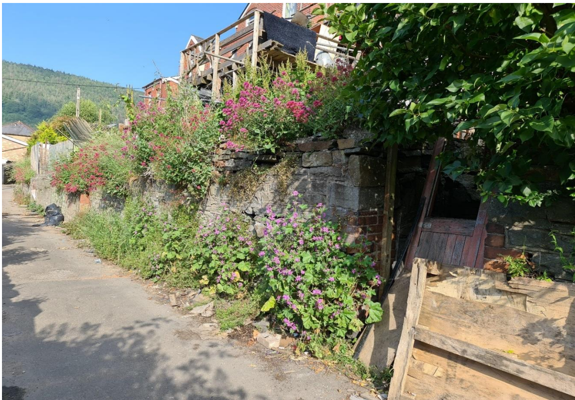
Examples of Rear Retaining Walls
